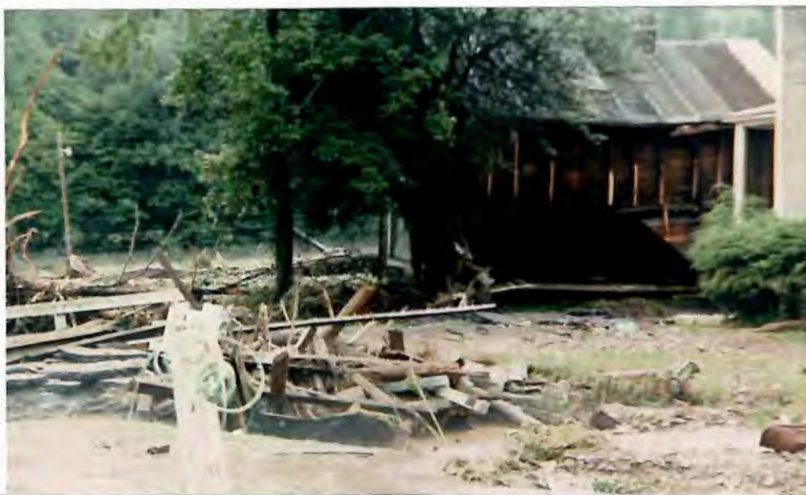
THE LARGE TREE PLANTED BY FORMER STORE KEEPER, I. D. LEYDIG KEPT THE DELAPIDATED POST OFFICE STRUCTURE AND THE FORMER MARTZ HOUSE FROM BEING SWEEPED FARTHER AWAY WITH THE RAGING FLOOD WATERS. NOTICE THE RUBISH IN THE CREEK.
